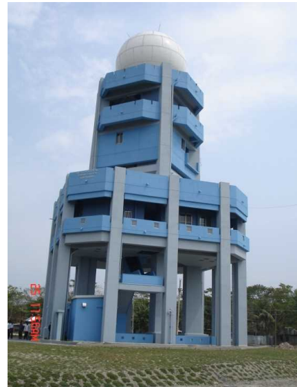
Khepupara Radar Station
