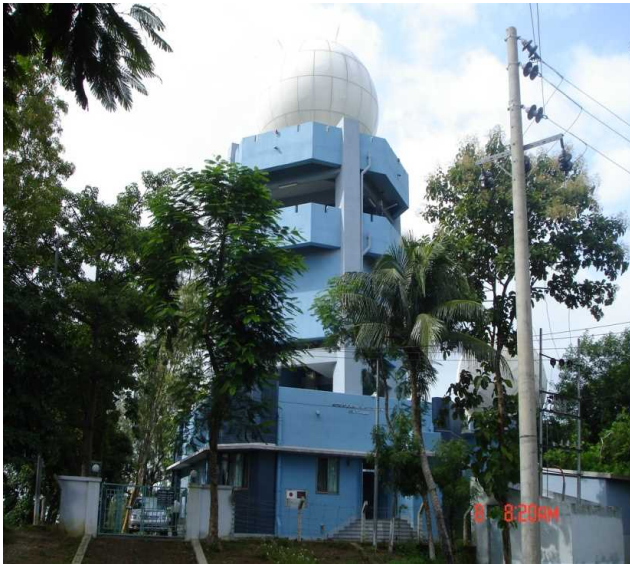
Cox'sbazar Radar Station
